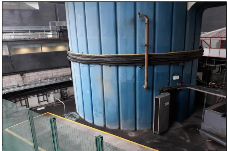
There is a diesel storage tank located in the south spiral core, which will require replacing and relocating including connection pipework etc. There are also a significant amount of extraction vents and other M&E installations supported by the spiral structure, therefore alternative supports would need to be erected to facilitate demolition.
